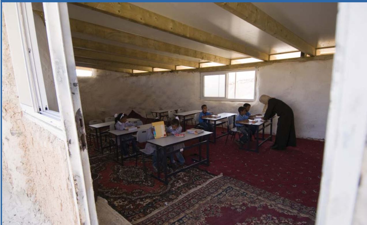
Al Khan al Ahmar school, included in the Area C Response Plan, serves Bedouin children in the Jerusalem governorate. It faces the threat of demolition due to the lack of a building permit. Photo by Patrick Zoll.
