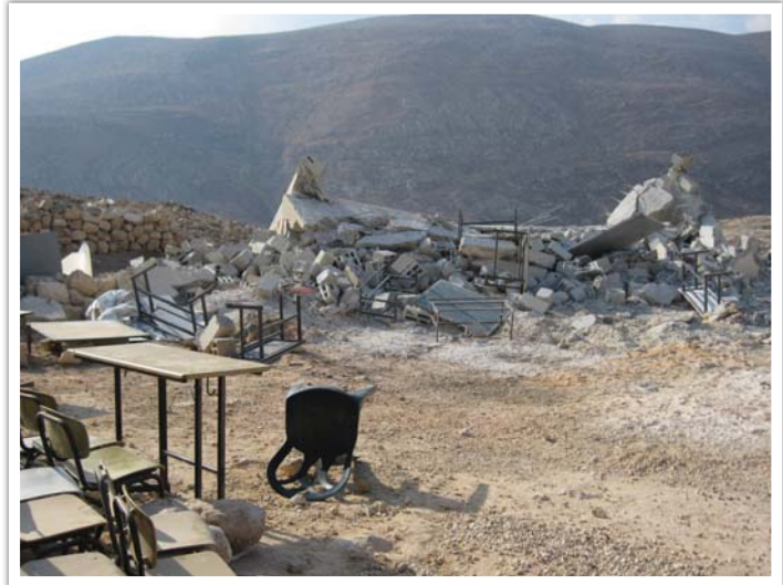
Remains of the Khirbet Tana school, demolished by Israeli forces in December 2010.
