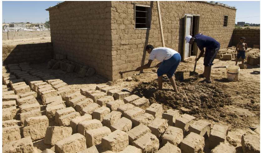
Gazans using mud bricks to reconstruct a home destroyed during the "Cast Lead" offensive. Photo by Patrick Zoll.
