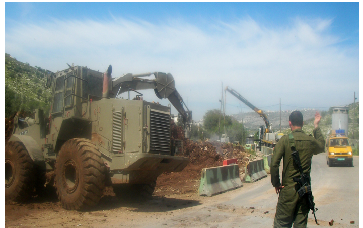
IDF Expansion of Enav checkpoint, Tulkarm. Photo taken in March 2009.
