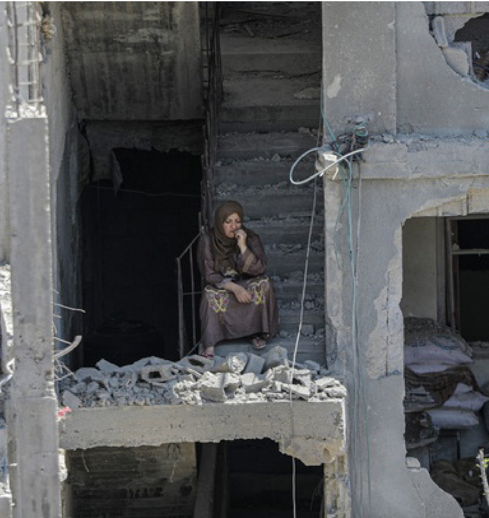
Destroyed homes- Beit Hanoun . © 2021 UNRWA Photo By Mohamed Hinnawi
