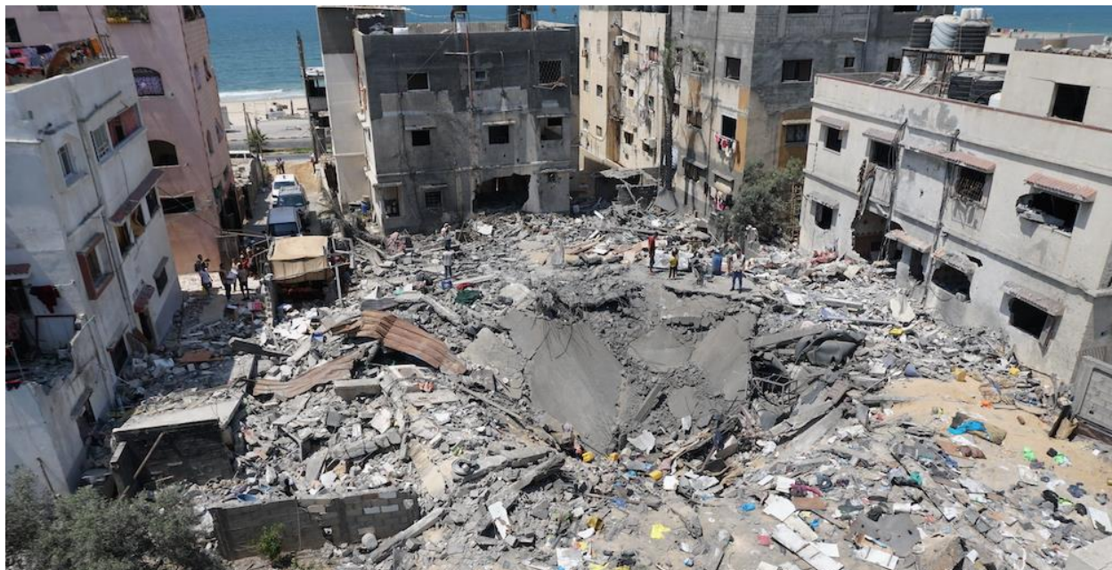
Destruction following the Israeli airstrike during the escalation in August 2022. © Photo by OCHA
